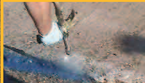
Aqualastic™ bridges cracks to accommodate expansion and contraction from freeze-thaw cycles unlike conventional caulk/joint fill products.
