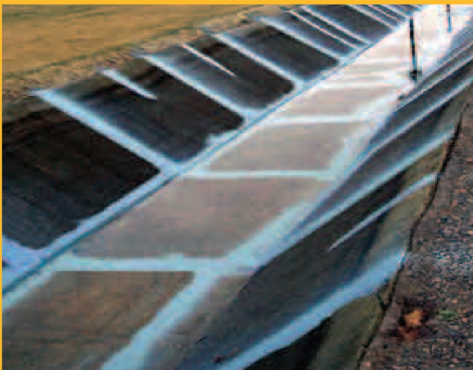
Aqualastic™ bridges cracks to accommodate expansion and contraction from freeze-thaw cycles unlike conventional caulk/joint fill products.
